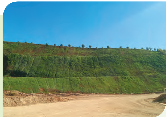
華潤水泥（鶴慶）有限公司礦山復綠 Ecological restoration to the mines of China Resources Cement (Heqing) Limited
