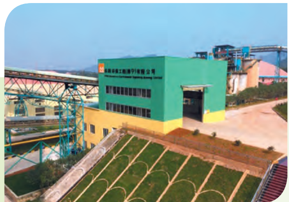
華潤環保工程（南寧）有限公司協同處置市政污泥示範項目 The demonstration project of urban sludge co-processing of China Resources Environmental Protection Engineering (Nanning) Company Limited
